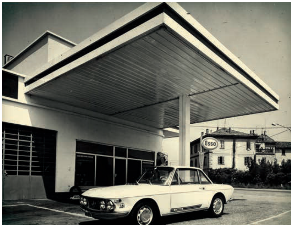
An elegant cantilever roof built with opaque corrugated Elyplast plates at an Italian gas station.
