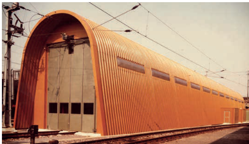
Railway carriages yard built with Elyplast.
