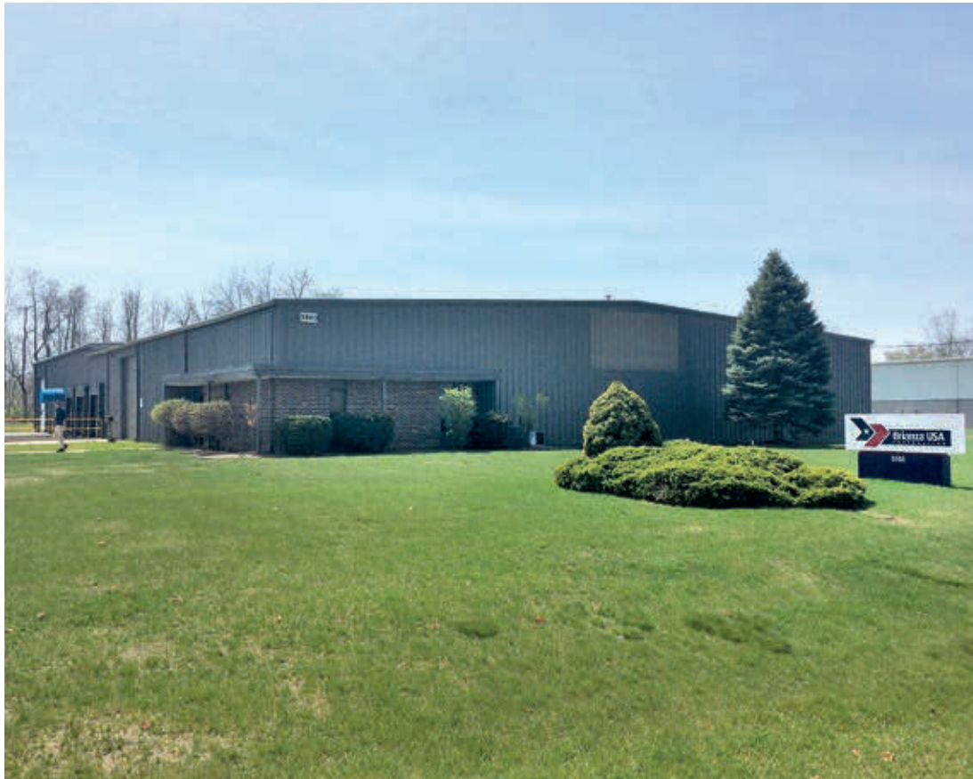
Brianza USA Corp., Elkhart, USA, international logistic and business centre
