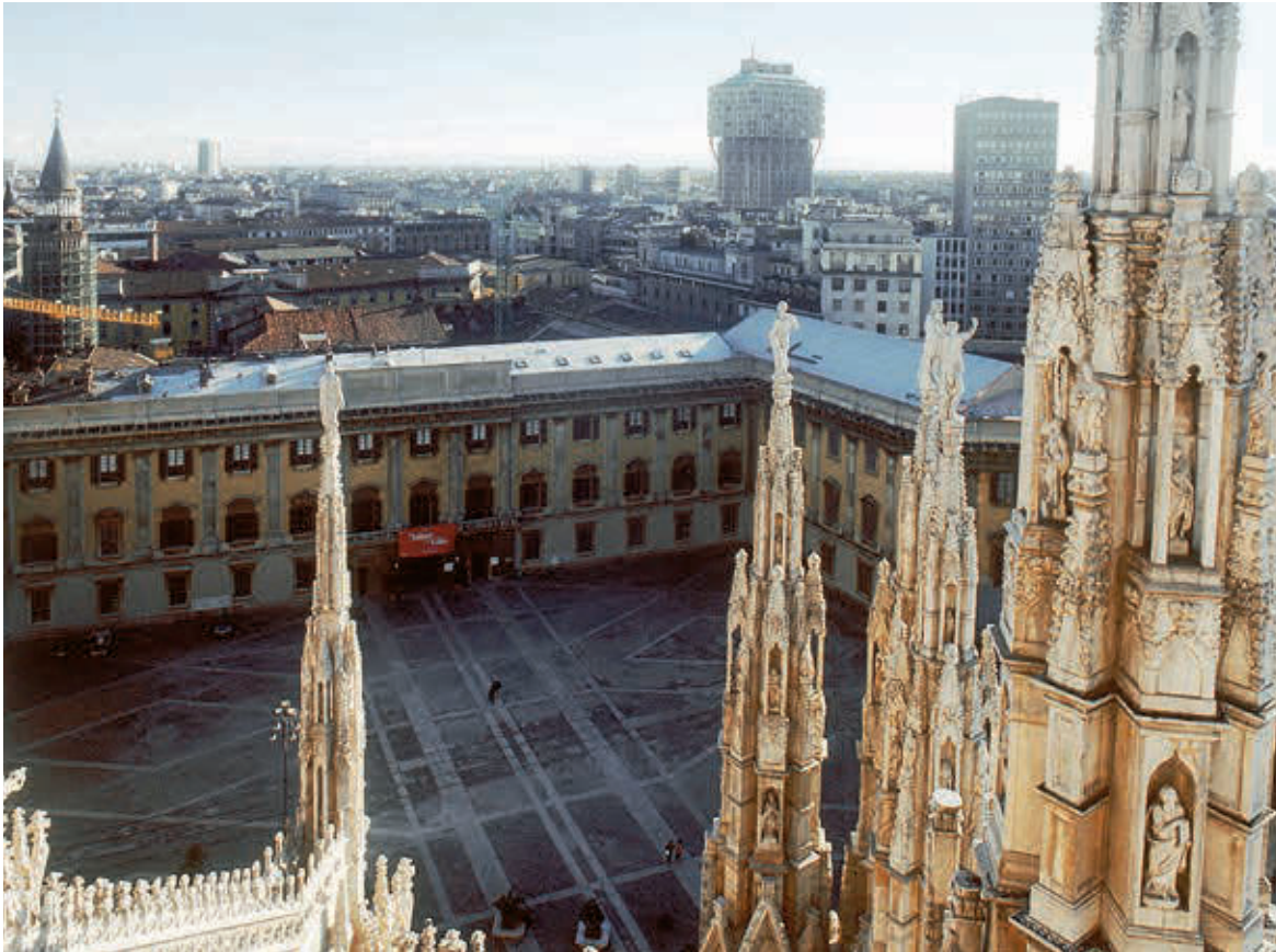
Milan - Isotec applied on the roofing of Palazzo Reale (Royal Palace).
