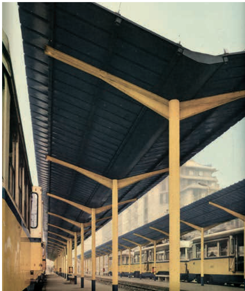
Suspended roofing built to cover the transit tracks of Milan's subway with Elyplast opaque coloured plates.
