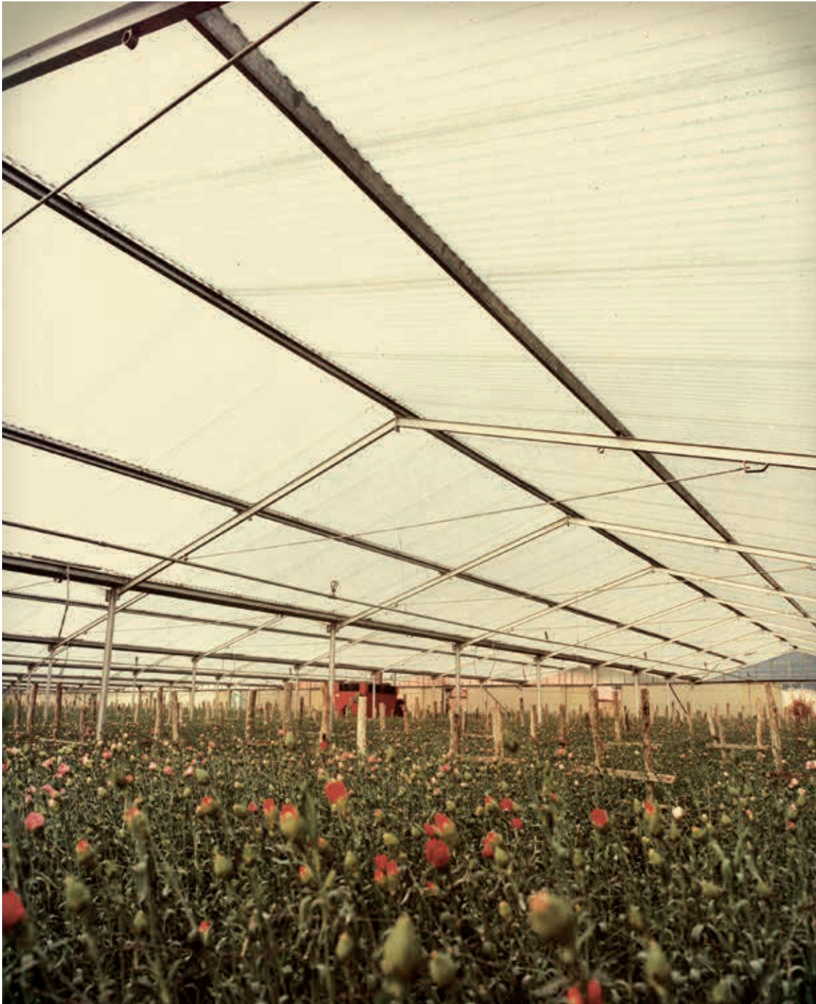
Elyplast corrugated translucent plates covering a greenhouse for the cultivation of flowers.
