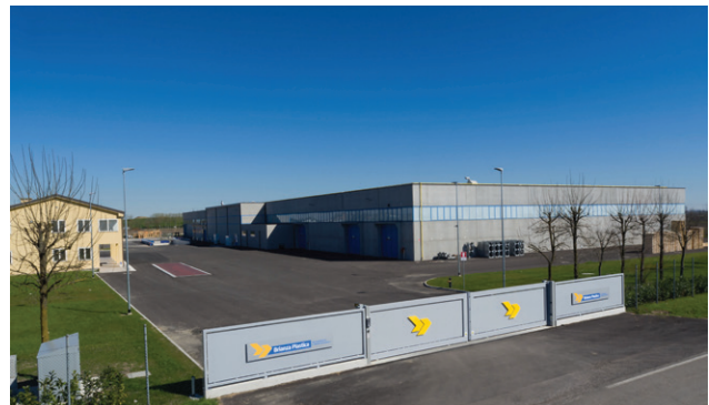
Brienza Plastica S.p.A. - Production site of Rovigo 2, Italy.
