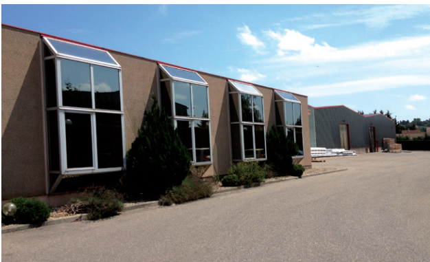
Plasti-Bat - Commercial warehouse of Diemoz, France.
